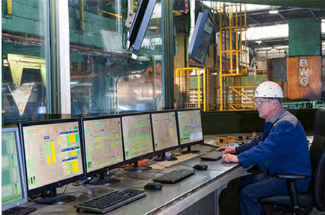
Reference: V7 control room
